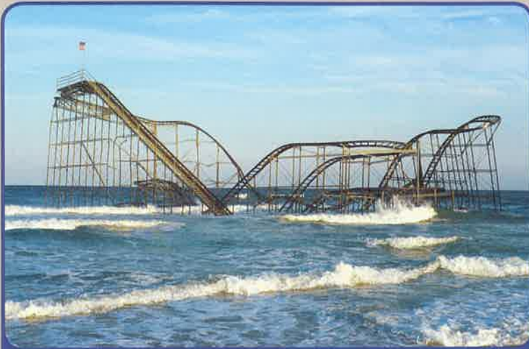
The Jet Star roller coaster fell into the ocean during Hurricane Sandy. The pier it was sitting on collapsed.
